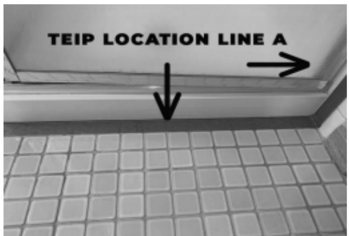
This will guarantee the prevention of the enamel from traveling under the masking plastic, and going on areas that are not to be refinished. It is also no problem if areas under the masking tape are not refinished. After the enamel solidifies, the tub will then be covered with silicone.
